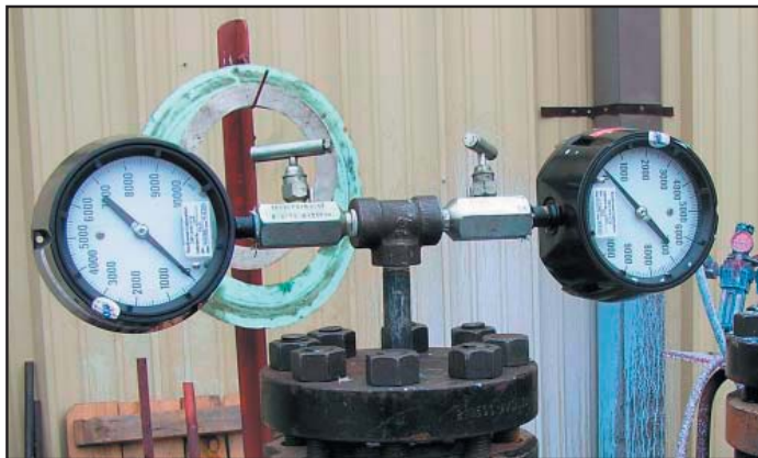
←← Pressure Gauges during testing
